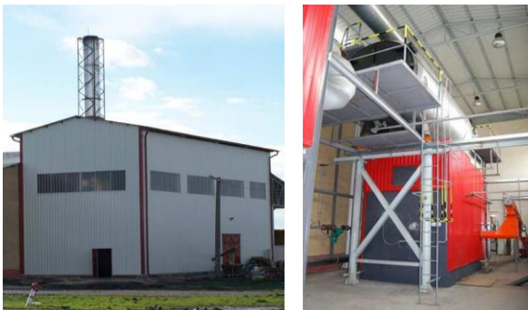
Fig.4 Boiler room for biomass combustion
