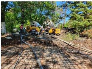
Photo 19 Deployment of two concrete pumps for simultaneous operation
