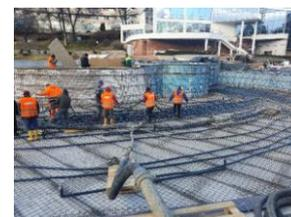
Photo 14 Piping for concrete horizontal transport
