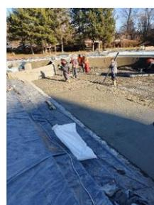
Photo 17 Bottom slab concrete casting
