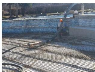
Photo 12 Walls and bottom slab steel mesh fixing
