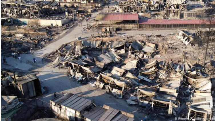
Fig. 3. Results of a fire due to overload of the electrical network in the modular town, Bosnia and Herzegovina [17].
