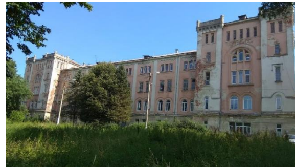
FIGURE 4. Castle of Count Stanislav Skarbek in the village of Zaklad, Mykolaiv district, Lviv region (author's photo)
