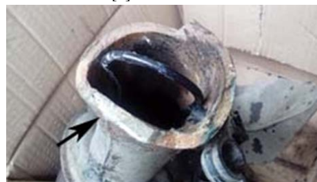
Figure 6 Deformed cross section of the broken sleeve
